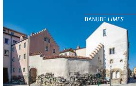
Above: Parts of the Roman wall at the north-eastern corner Below: The "document Legionslagermauer" at Dachauplatz
